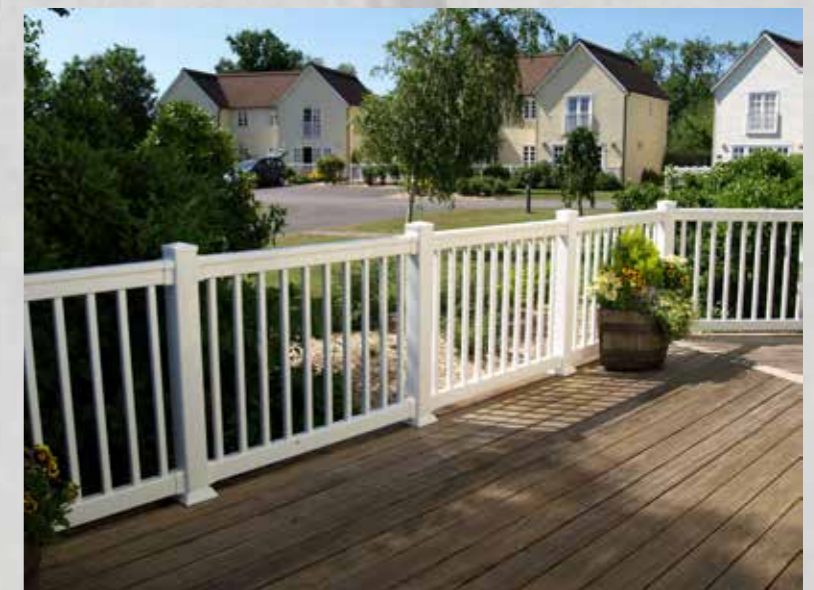
Balustrade style fencing
