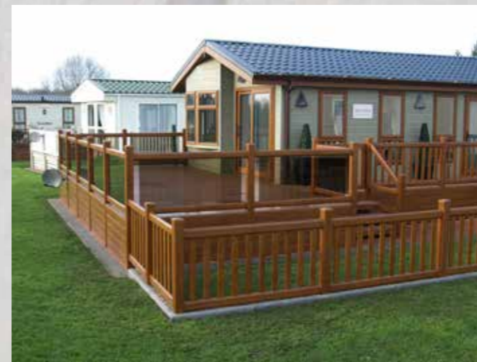
Golden Oak balustrade with additional fencing area
