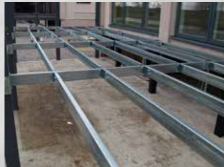
Galvanised steel sub-frame
