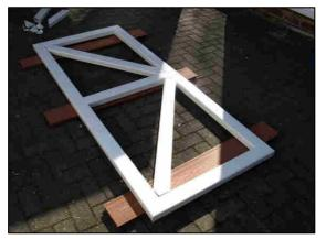
The image shows how the gate frame should now look with the cross braces in place.
