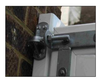
The 2 hooks can now be fixed to the hanging post using the supplied self drilling tech screws. It will be necessary to position the gate frame next to the post to determine the position of the gate hooks. Fasten both hooks to the hanging post making sure they are fixed into the steel inside the post.
